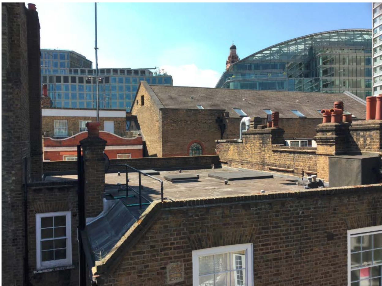
Roof of 12-14 Wilfred Street (application site) as viewed from rear
